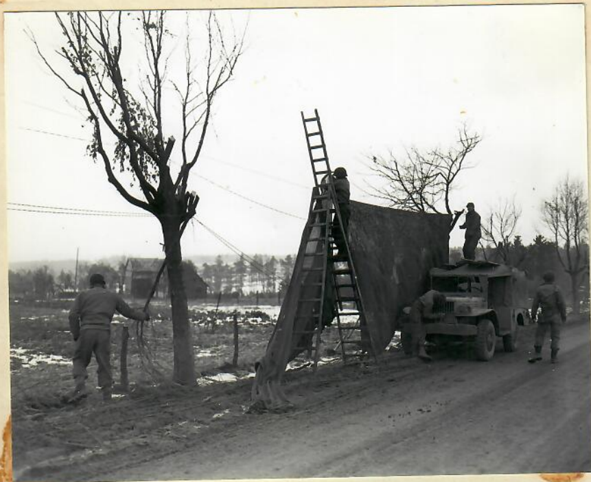
3rd and 4th Platoons of Company C constructing a road screen of shrimp nets, 1\frac{1}{2} mi. long. This screen concealed convoy traffic on a supply road under enemy observation.
