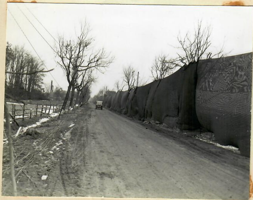
3rd and 4th Platoons of Company C constructing a road screen of shrimp nets, 1\frac{1}{2} mi. long. This screen concealed convoy traffic on a supply road under enemy observation.
