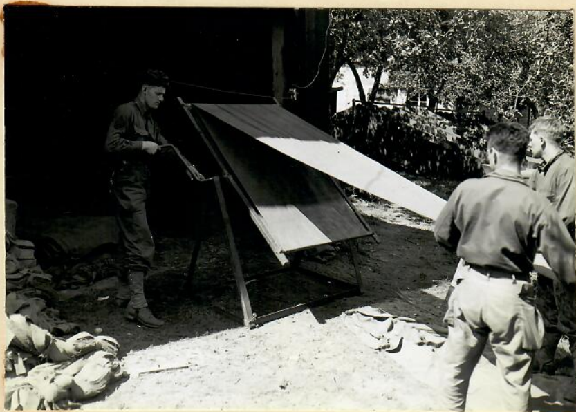
A device for folding dyed burlap in 5 foot lengths.
