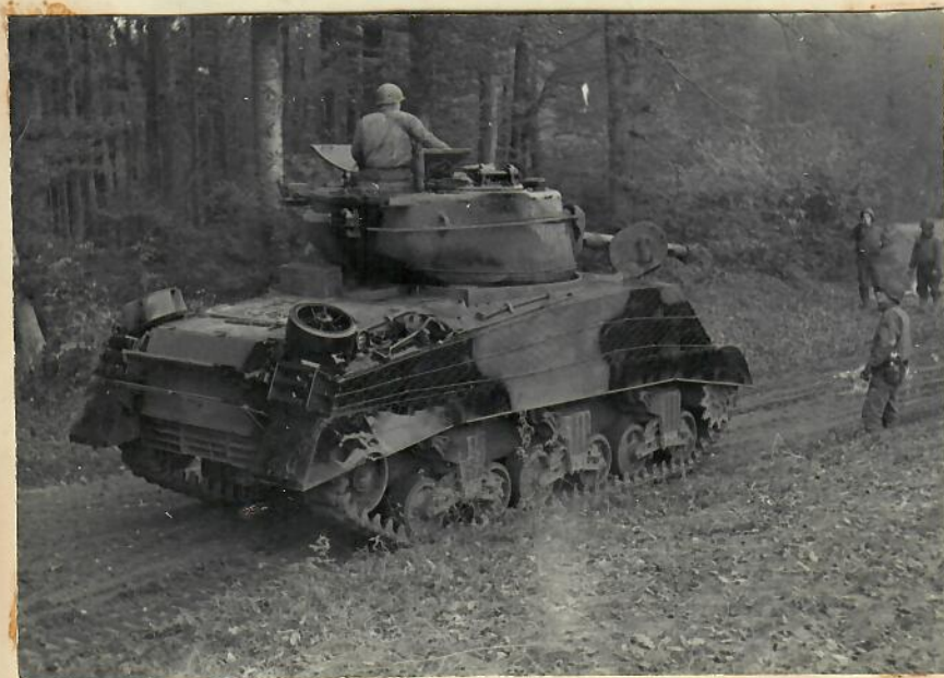
Sommerfeld mat applied to a tank, after which pattern painting is applied. Assistance and supervision of the work was provided by Cos B and D of the Bn.
